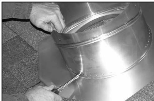
2. After turning bottom of elbow clockwise to align roof pitch number with indicator line on flashing. Place 3 short screws through holes that line up with predrilled holes in base.
