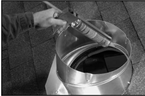
8. Seal all seams and nails with roofing cement.
