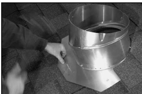
5. Slide top half of flashing under shingles. Secure with nails.
