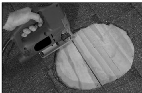
4. Cut hole as marked. Seal around top and sides with roofing cement
