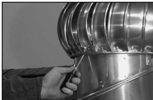
10. After installing check to see that whirlybird turns freely. In transportation it may have shifted slightly. If necessary, minor adjustment may be made by gently prying lowest point of turbine upward to remove any wobble.
