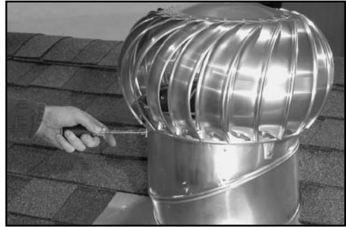
9. Position whirlybird on the base. Line up the predrilled holes in the brackets and base and fasten with long sheet metal screws.
