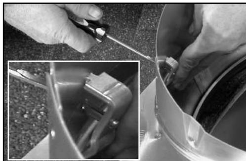
7. Place locking clamp across seam and tighten as shown, with machine screw.
