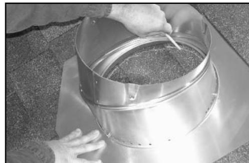
3. Using back of this page determine placement of turbine(s). Locate base opening between rafters and mark hole(s) to be cut. Locate rafters by tapping roof.
