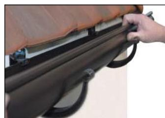
Place the gutters on the support brackets.
