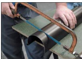
Saw the gutters with a hacksaw to the necessary length.
