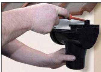
Install the connectors and the outlets while descending 3mm.
