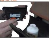
Glue the stopend to the gutter, use PVC glue.
