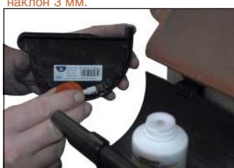
Glue the stopend to the gutter, use PVC glue.
