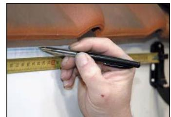
Place the necessary support brackets with a distance of  $\pm$  33cm.
