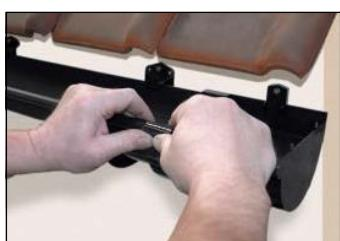
Click the gutter into the connector and outlet.
