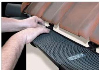
Put the gutter screen on the gutter.
