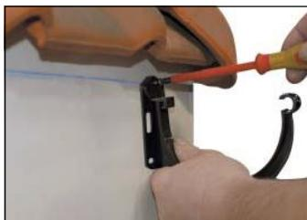
Determine and measure the line / direction.
