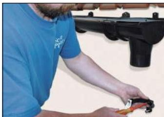
Install the fixo in the direction of the drainpipes.
