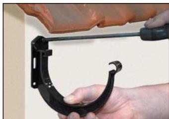
Attach the support brackets, while descending 3 mm in the direction of the drain-pipes.
