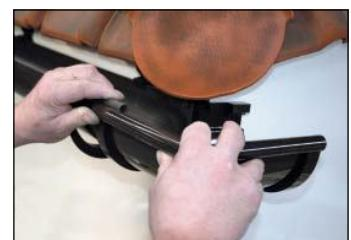
Before final installation, connect the gutter to the angle.
